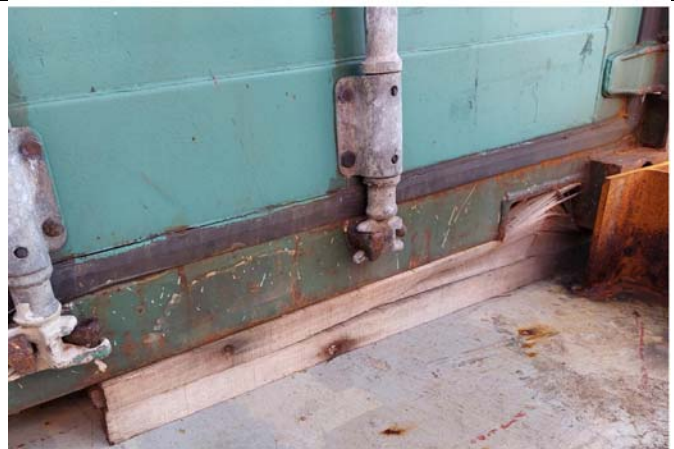
Wooden dunnage used for weight distribution
